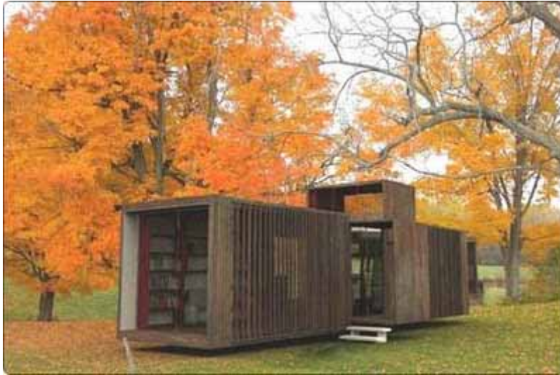
Drop House de D3 Architectes
